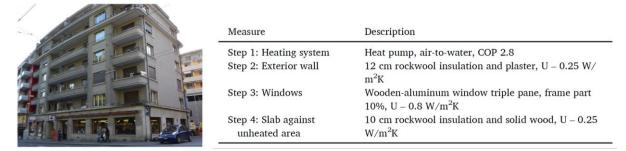
Figure 21: Building for case study 1. Figure 22: Measures applied following each iteration of the sensitivity analysis.
